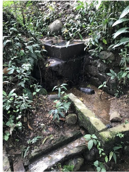
Figure 3: Main Water Source- Water Spring, Filter Chamber and Drains
