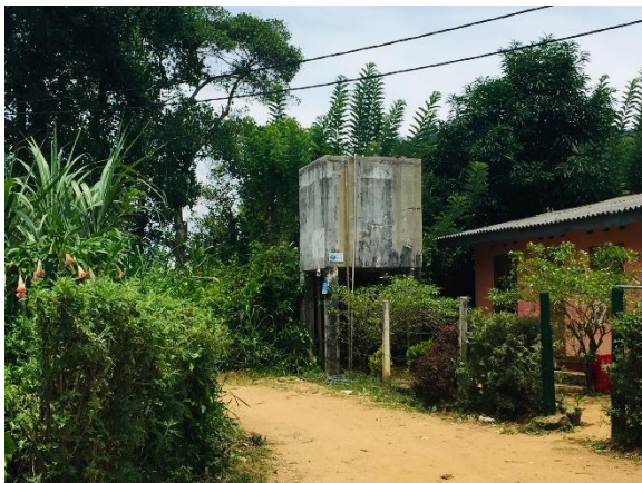
Figure 2: Two water supply systems in Mahatenna
